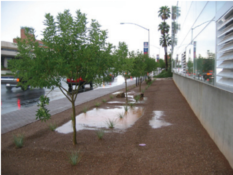
Micro-basins collect and hold extra water for plants during a rain event in front of the new College of Architecture and Landscape Architecture Building on the University of Arizona campus.
