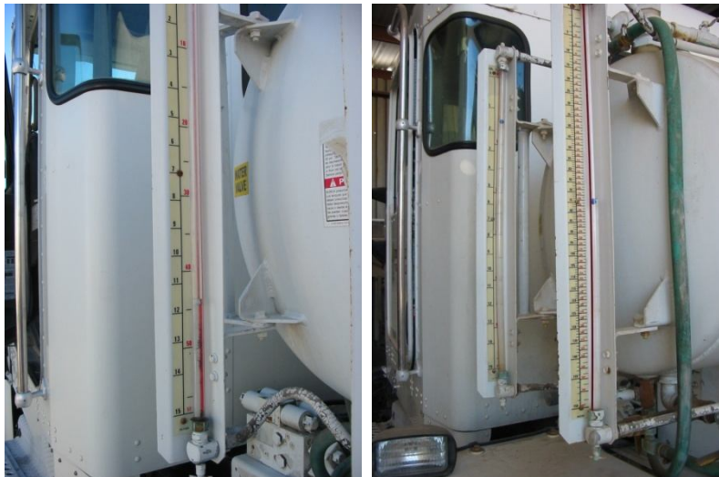
Figure 3: Legible Water Site Gauges
